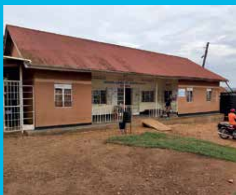
Figure 1: Health Centre II-Current.
